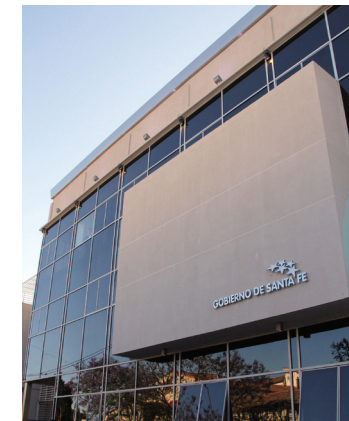
Santa Fe Data Processing Centre
